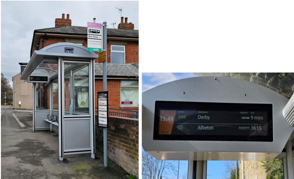
Figure 13: Newly installed RTI
