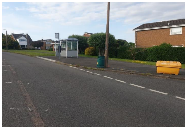
Figure 5: Corridor 43, after improvements
