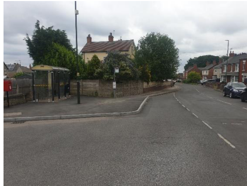
Figure 9: Corridor 77, after improvements
