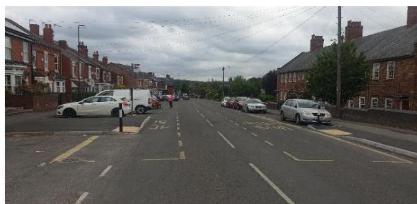
Figure 7: Corridor 77, after improvements
