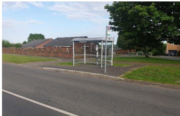
Figure 3: Corridor 43, after improvements
